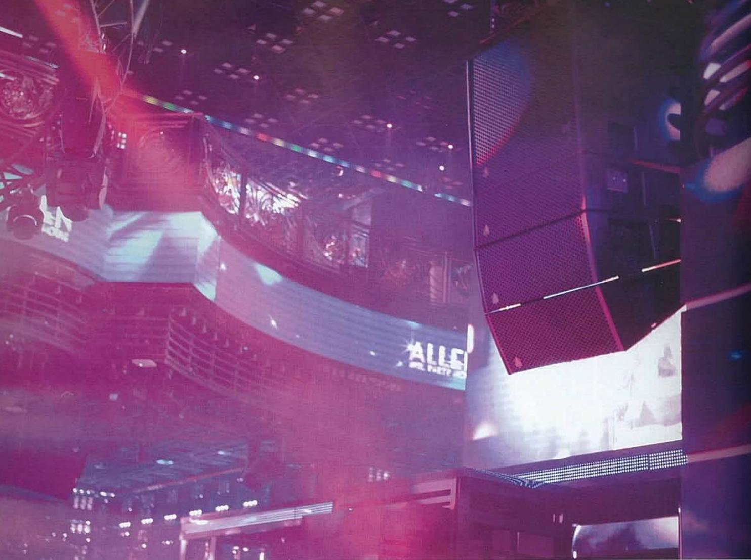
to ensure maximum average SPL of 130dB, while ensuring  $\pm 3$ dB disparity.
